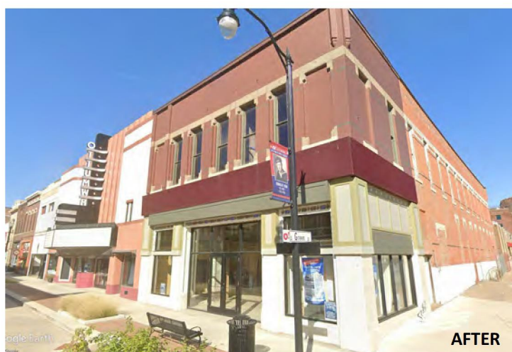
Downtown Ottumwa has taken tremendous steps to encourage the renovation and restoration of properties and storefronts throughout the district.
