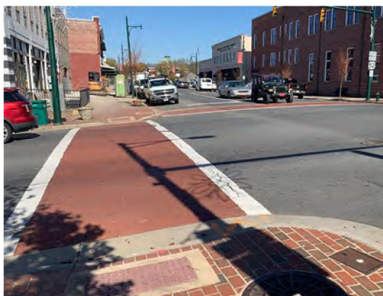
The white stripe on either side of the crosswalk adds definition and highlights the pavers.
