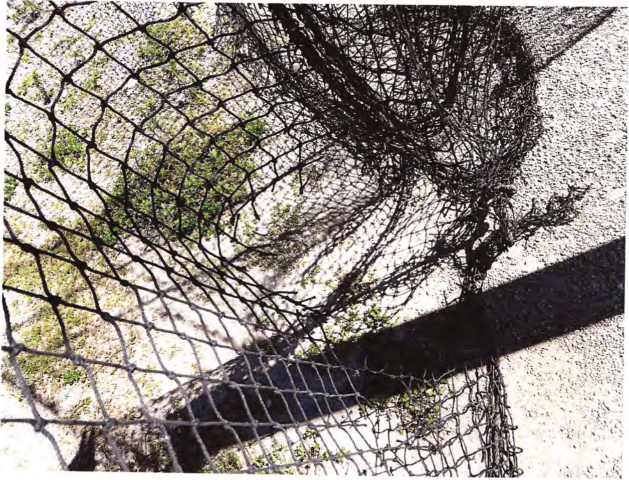
Another batting cage pic, with upclose look at hole in netting.
