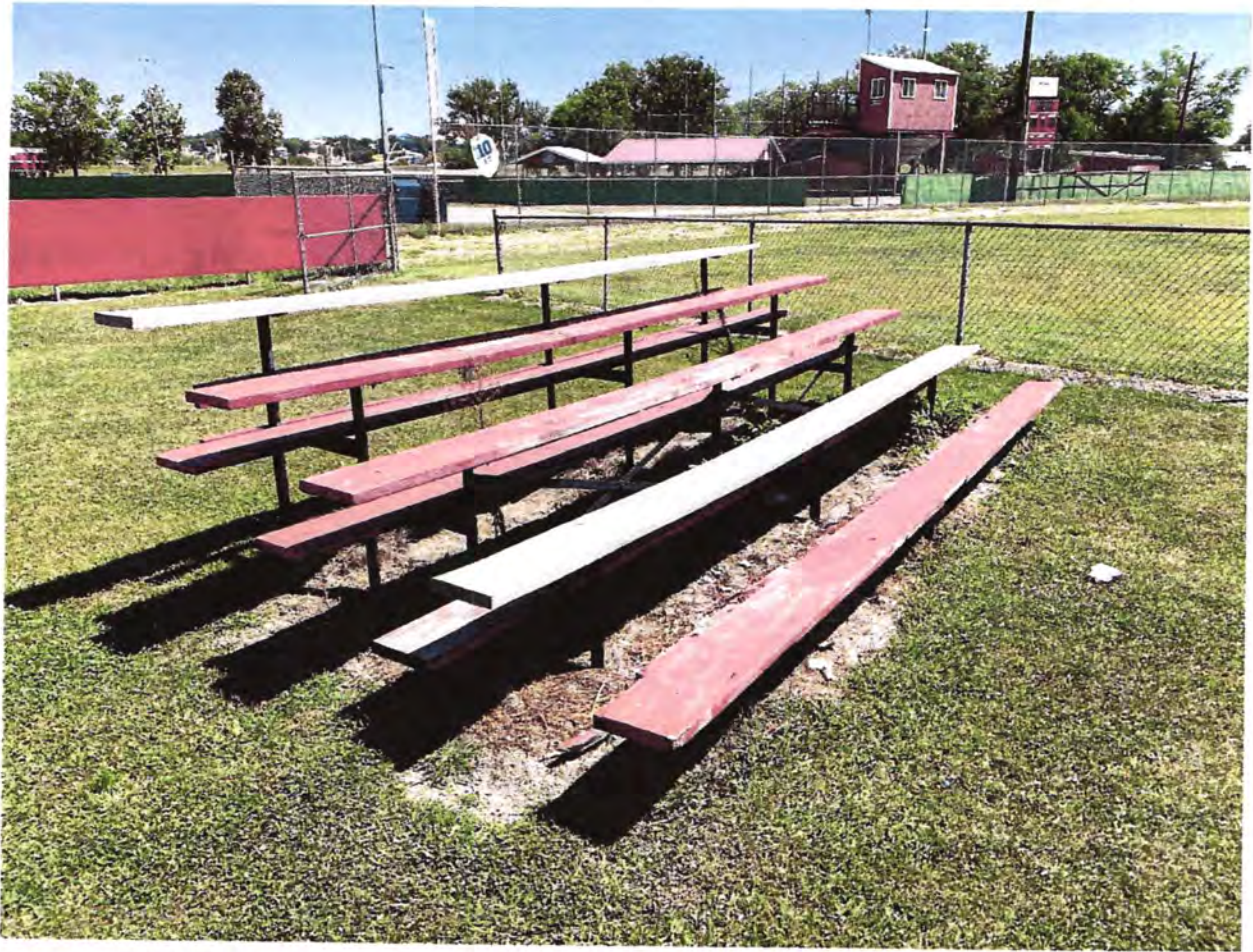
Replace boards and paint
