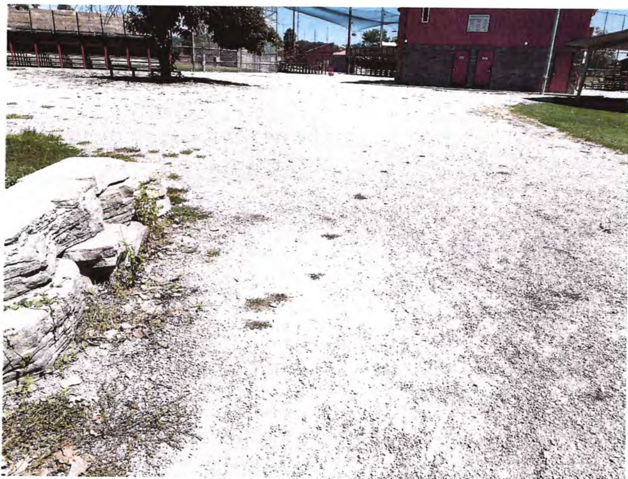
Additional gravel and weed control
