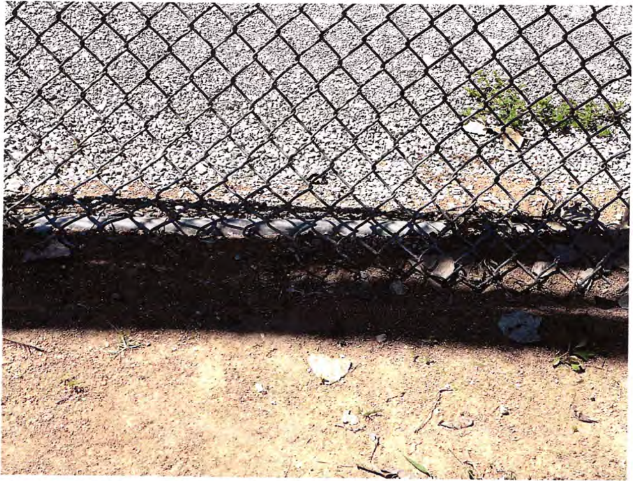
Closer look at back stop fencing curled up at bottom.
